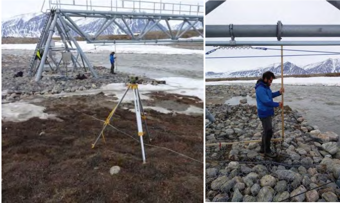
Figure 56: Lineup for levelling of the hoist trolley
