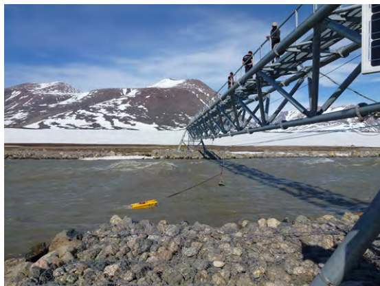
Figure 49: Discharge measurements are performed along the hoist trolley. Qliner is attached to the steel wire.
