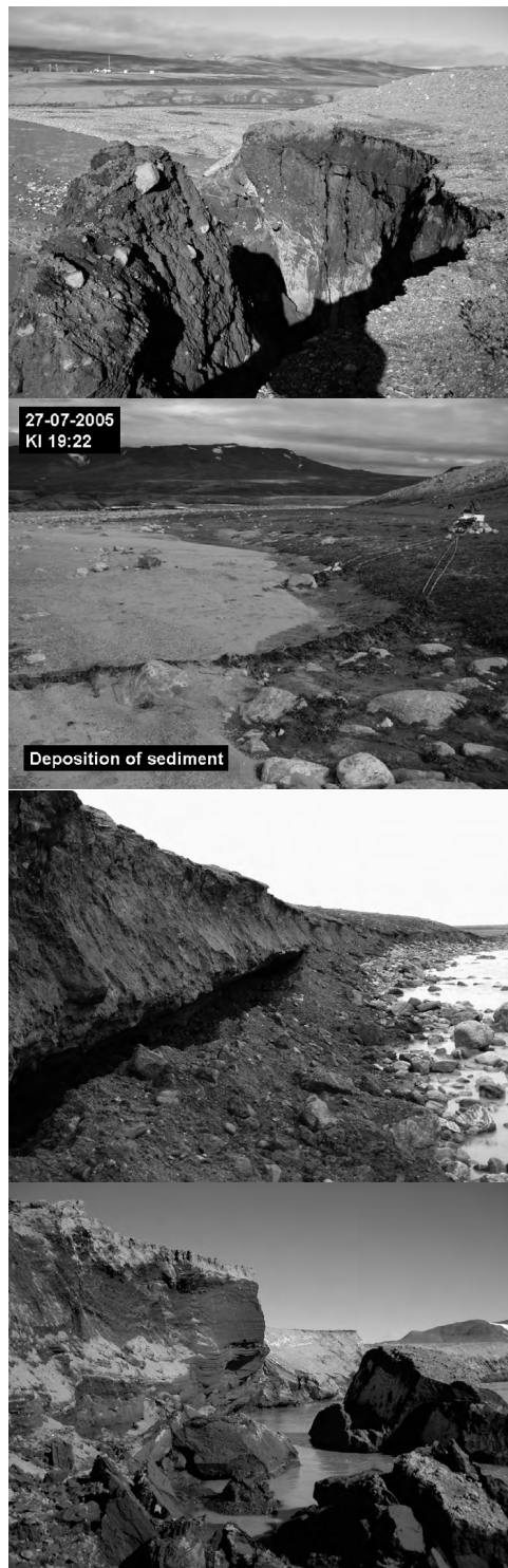
Fig. 2.19. Photos showing erosion along Zackenbergelven and at the delta cliff as a response of the flood 25 July.
