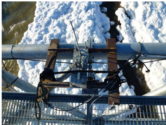
Figure 43: Metal frame for installation of OBS, diver and conductivity sensor
