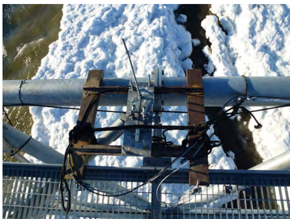
Figure 46: Metal frame for installation of OBS, diver and conductivity sensor
