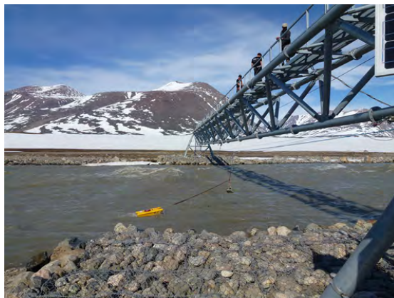
Figure 48: Discharge measurements are performed along the hoist trolley. Q.liner is attached to the steel wire.
