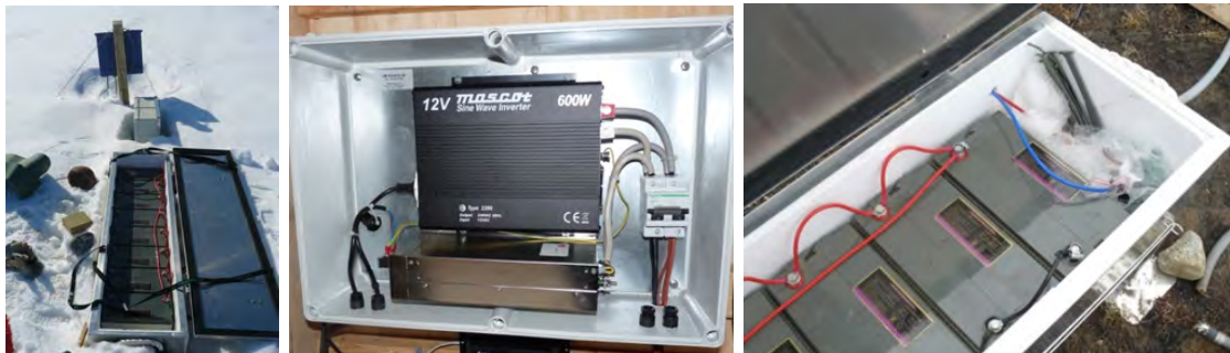
Figure 76: The battery box (left). A look into the transformer box, inside the hut (mid). Power cable from the instrument box enters the battery box in the southern end –the red and blue cable are connected to plus and minus on the last battery in the row.
